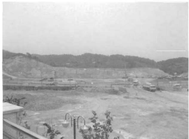
Fig.8 Surface Structures Site under Grading
